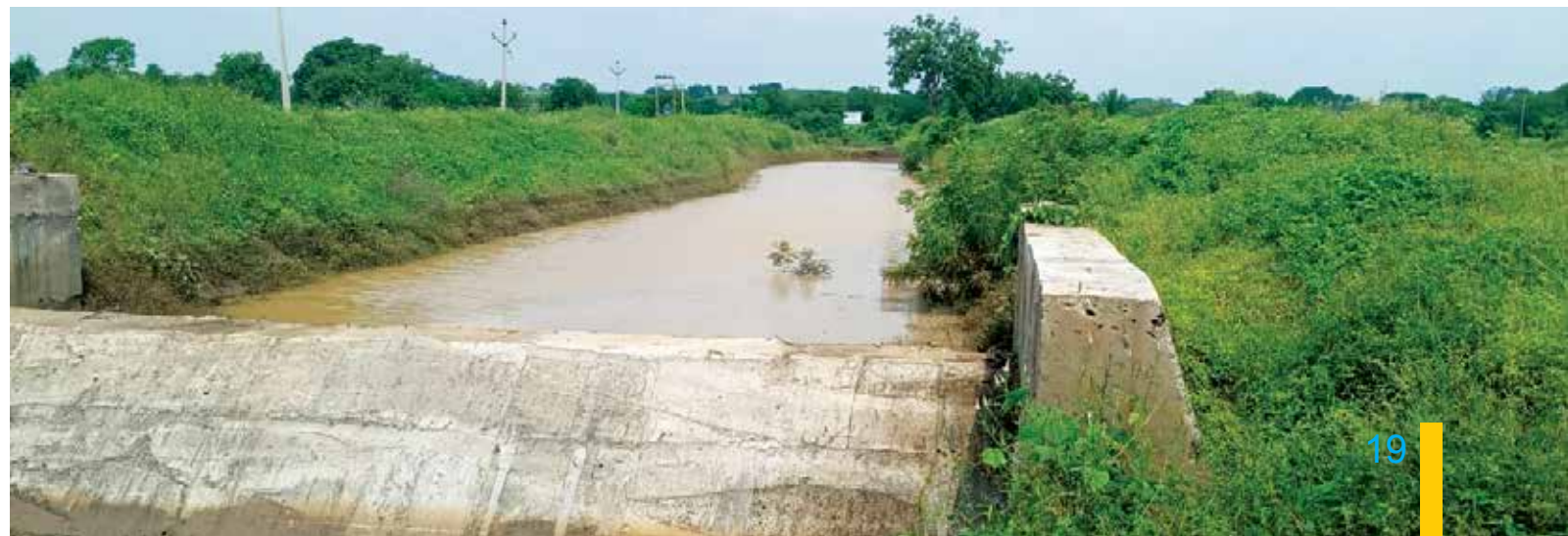
Cement Nala Bund (CNB) at Sugaon, Beed, Maharashtra
