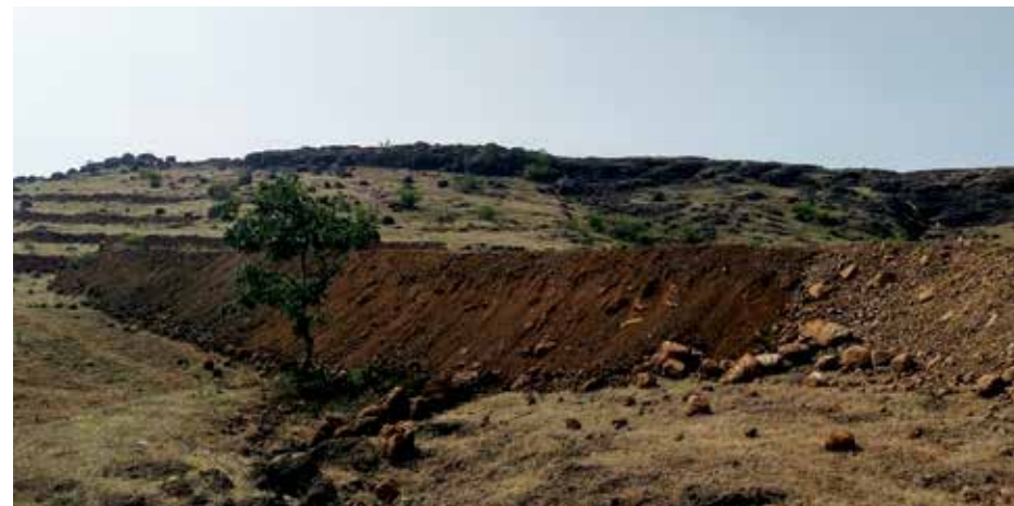
Earthen Nala Bund (ENB) at Ujjainpuri, Jalna, Maharashtra
