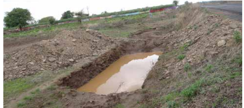
Water Accumulating Deep Trench (WADT), Radi, Beed, Maharashtra
