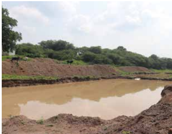
De-silted percolation tank, Roshangaon, Jalna, Maharashtra
