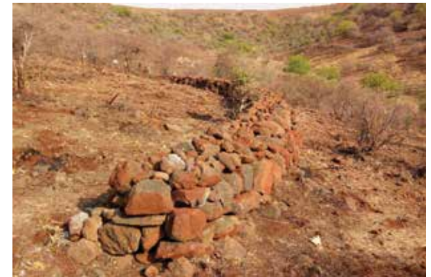
STONE BUNDING (SB) – These serve the same purpose as CCTs and are also constructed along the contour lines. In areas with hard strata and low soil depth where trenches can't be dug, small loose stones are stacked to form a bund.
