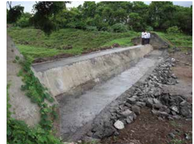
Cement Nala Bund, Khadgaon, Aurangabad, Maharashtra
